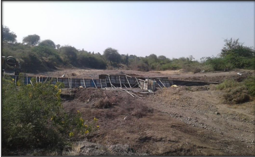
Picture:2 During progress work of Check dam
