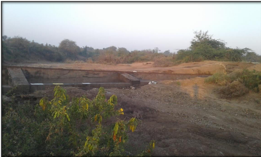
Picture-3 Completed Check dam
